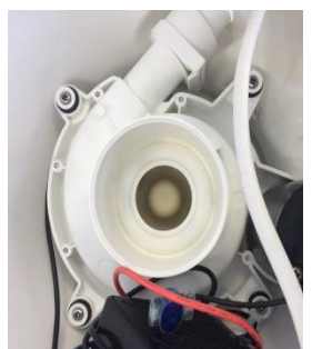
14. Replace waste pump
